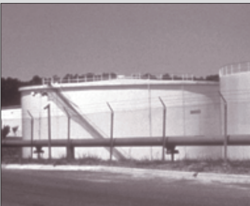
Chemical storage tank
